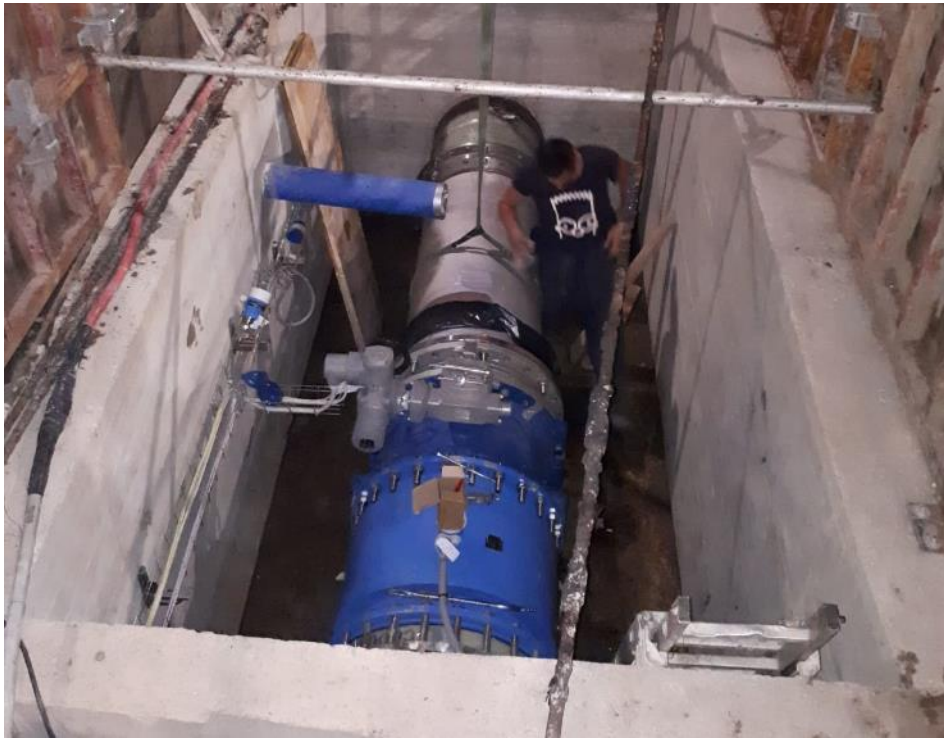
Connection works in a service chamber
