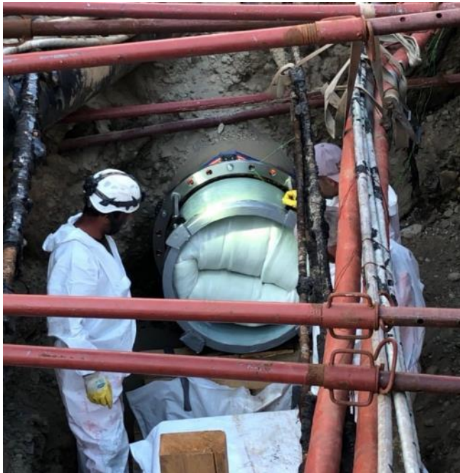
Pressure hose liner of classes A, B, C in acc. with EN ISO 11295
