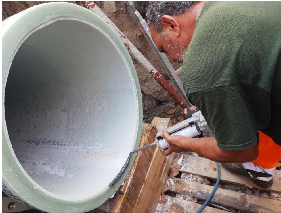
Sealing of the cutting edge
