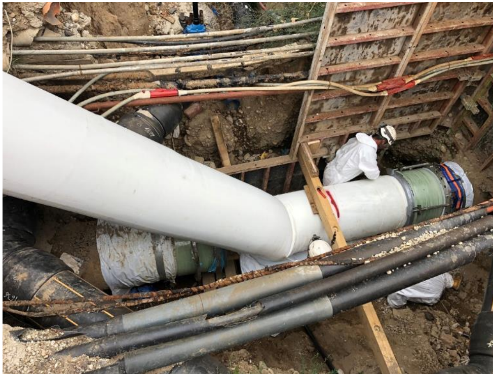
Installation of BlueLiner (Starting point)
